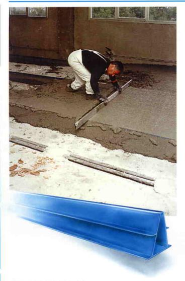
PVC guide to create castings with Politerm. Expansion joint for floors
